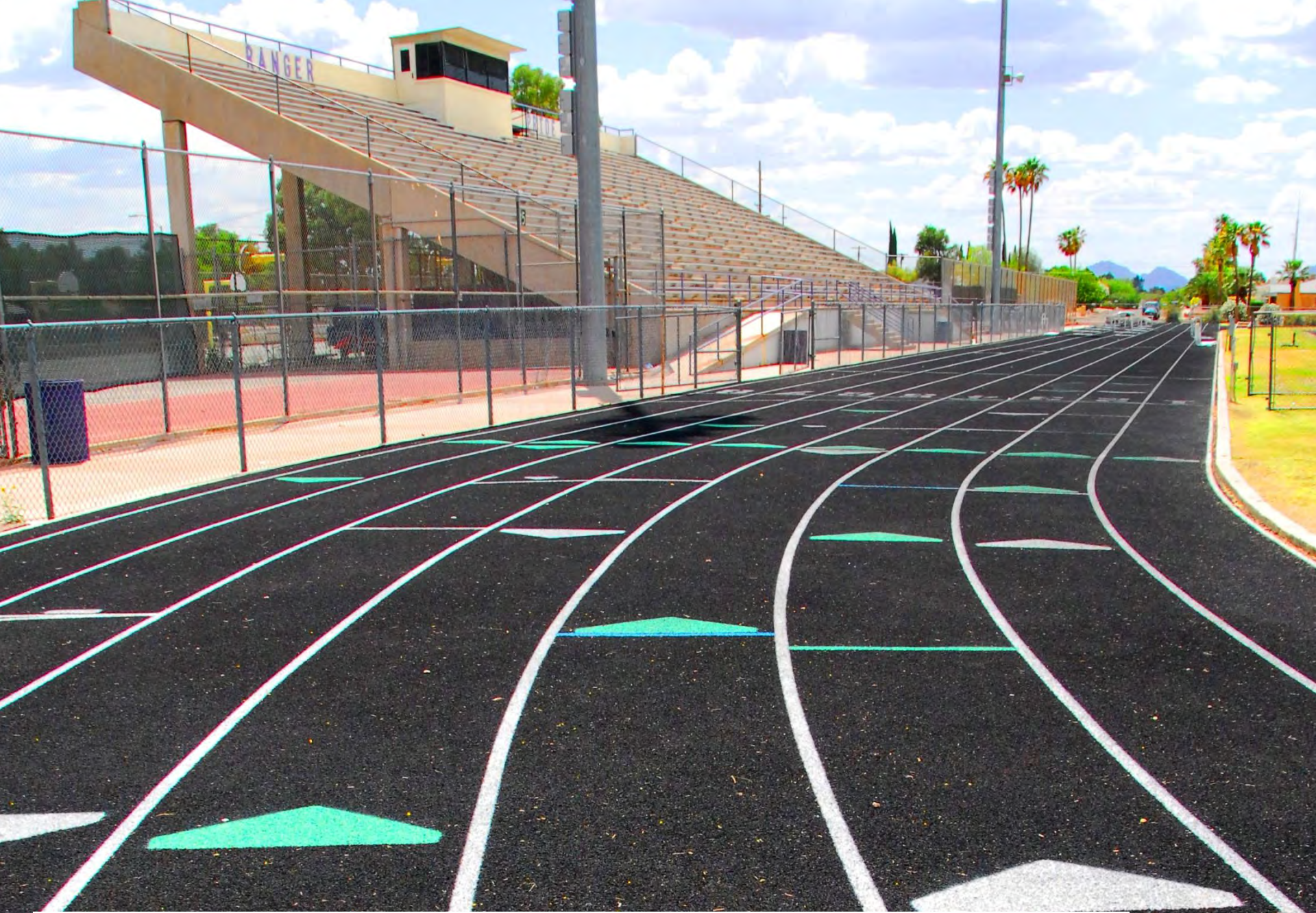
Rincon High School Track Renovations
