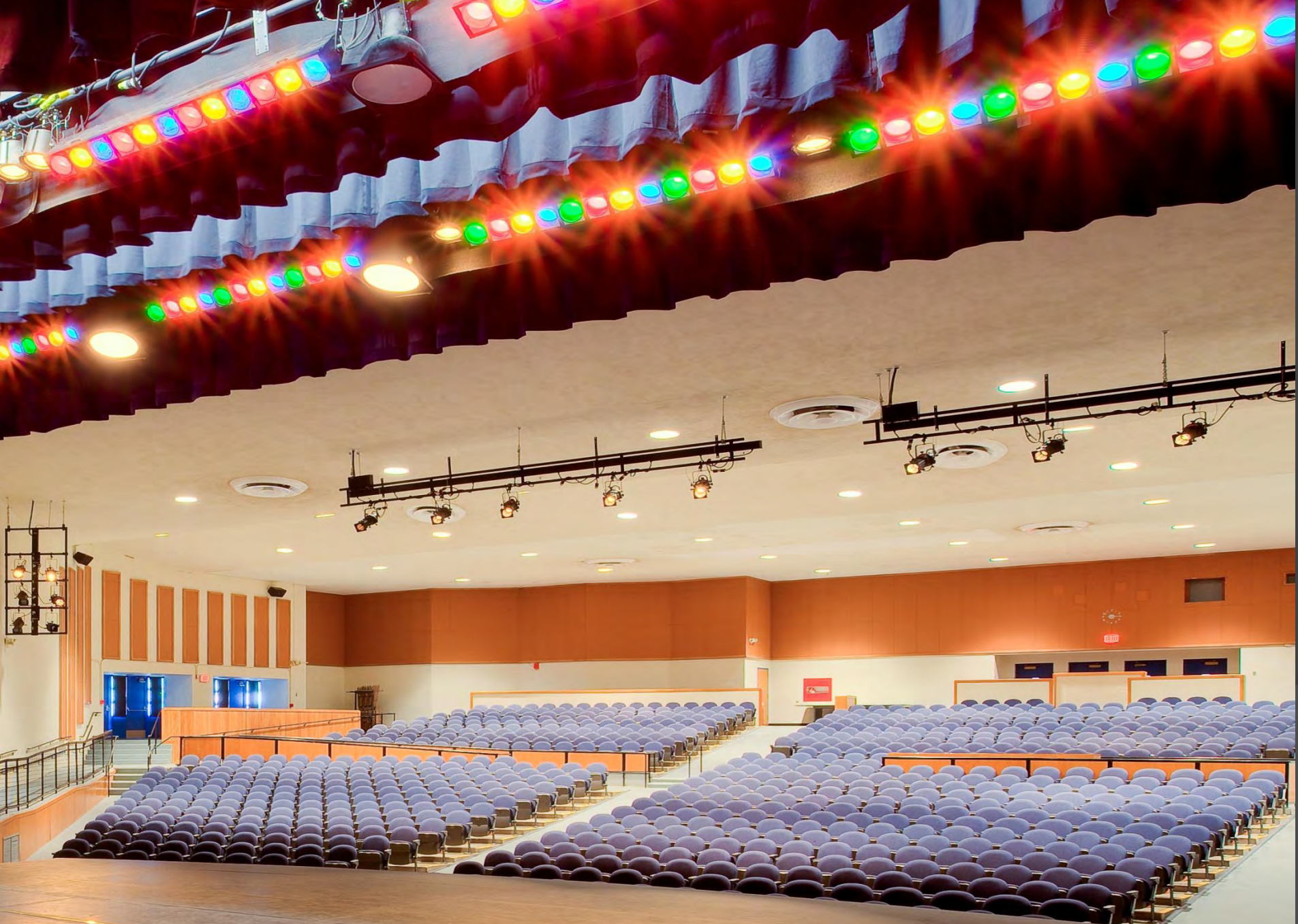
Palo Verde High Magnet School Fine Arts Renovations
