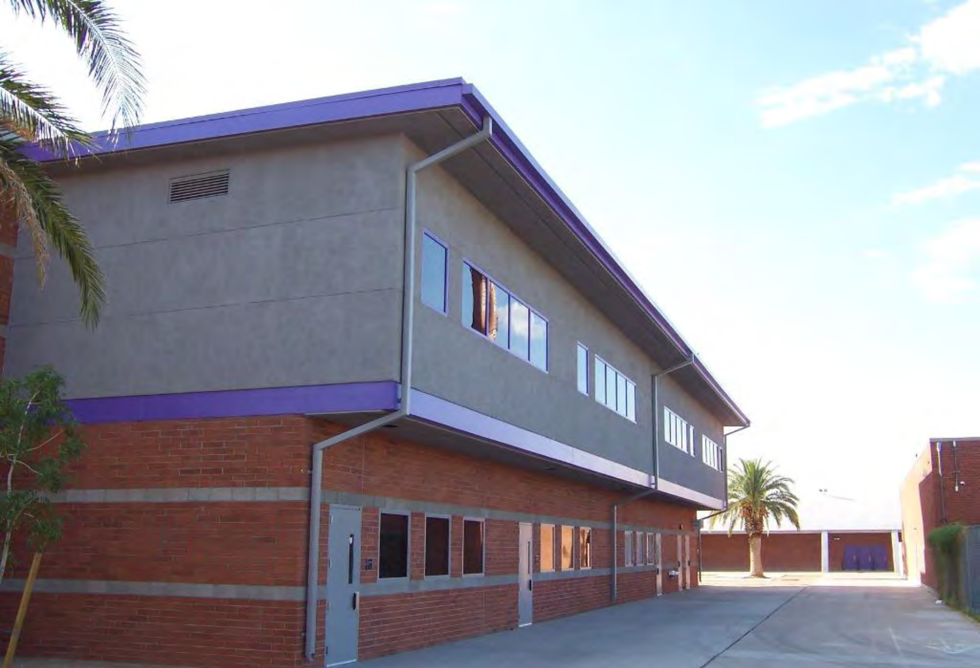
Rincon / University High Schools Classroom Addition
